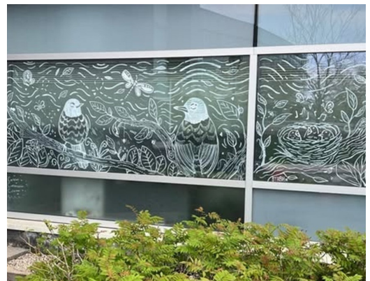
FIGURE 13. Window treatments at Carleton University help birds see glass and prevent window collisions. Photo: Safe Wings volunteer.
