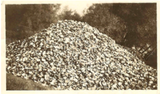
1 The Clam Shell Pile (original picture)
