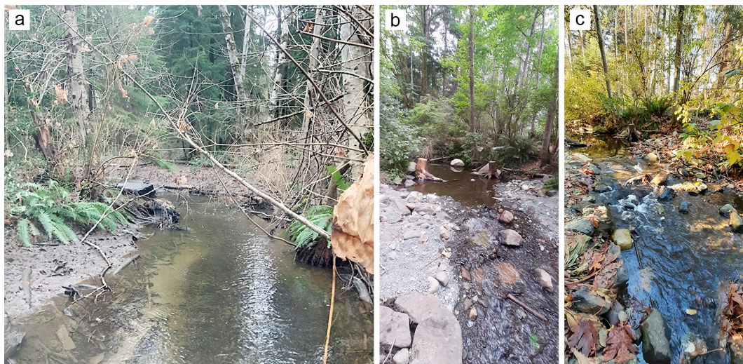
FIGURE 1. Arden Creek stream restoration for the Western Brook Lamprey ( Lampetra richardsoni ), Morrison Creek population at the most downstream riffle near the confluence with Morrison Creek. a. pre-restoration, b. immediately after riffle installation, and c. one year post-restoration. Photos: Joy Wade and Paul Grant.
