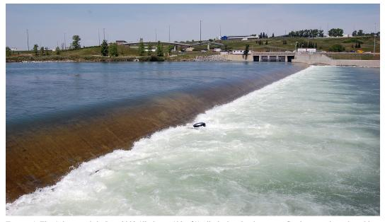
**FIGURE 1.** The Calgary weir in June 2009 (discharge 109 m<sup>3</sup>/s), displaying the river water flowing over the weir and into the hazardous hydraulic recirculation zone, with trapped sticks and a wheel. The structure on the far side allows offstream diversion into an irrigation canal. This system was subsequently modified with the Harvie Passage to produce safer paddling channels. Photo: Stewart Rood.
