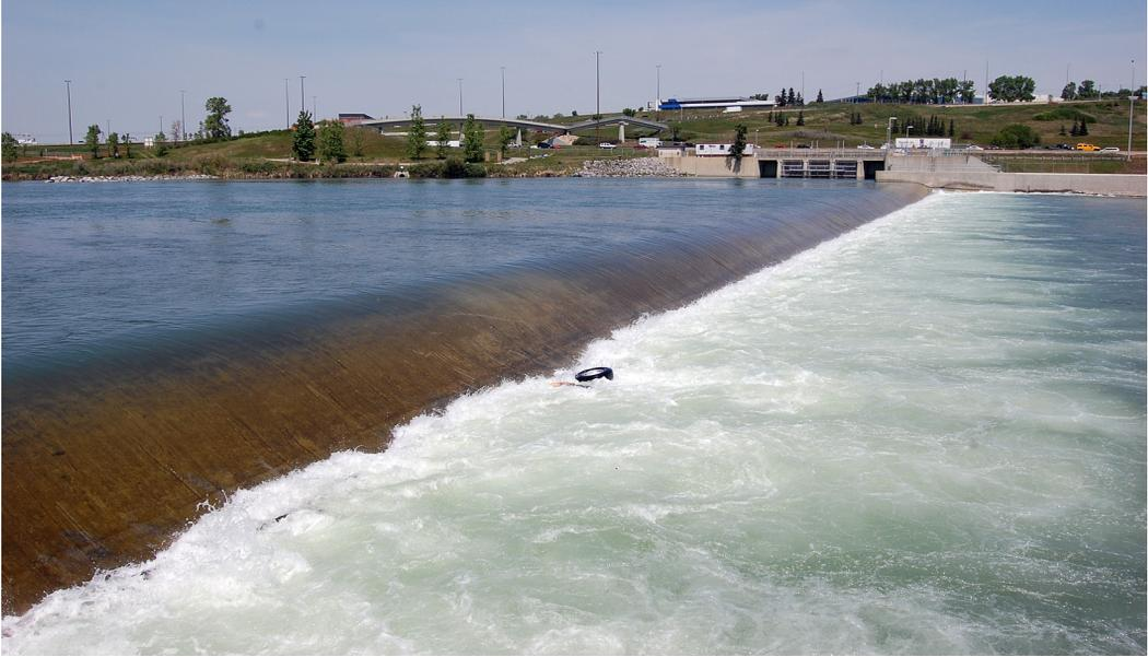
**FIGURE 1.** The Calgary weir in June 2009 (discharge  $109 \text{ m}^3/\text{s}$ ), displaying the river water flowing over the weir and into the hazardous hydraulic recirculation zone, with trapped sticks and a wheel. The structure on the far side allows offstream diversion into an irrigation canal. This system was subsequently modified with the Harvie Passage to produce safer paddling channels. Photo: Stewart Road.
